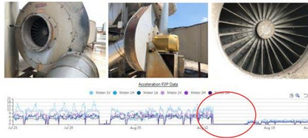
Fig. 5. Example of vibration data predicting a failure [5]
