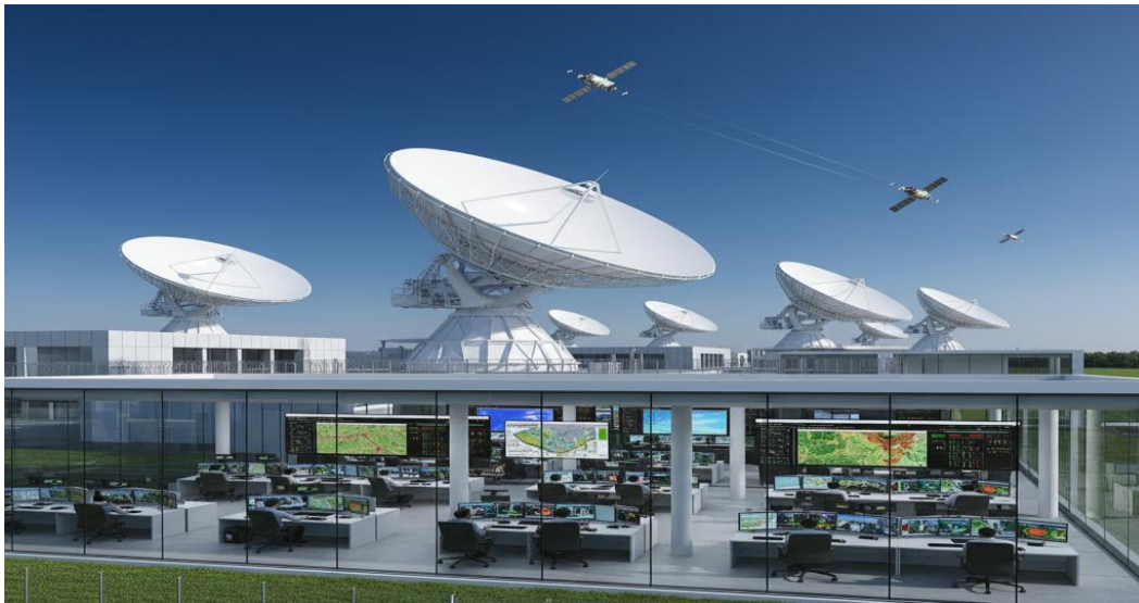
Figure 3: National Remote Sensing Center satellite ground station at Shadnagar, Hyderabad
